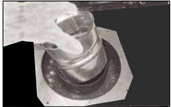
Figure 8.2 Remove the inner collar adapter.
